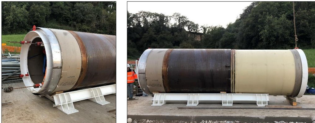
Figure 8 – View of the jacks and dywidag bars (left) and IJS assembled laying on the tracks (right)
